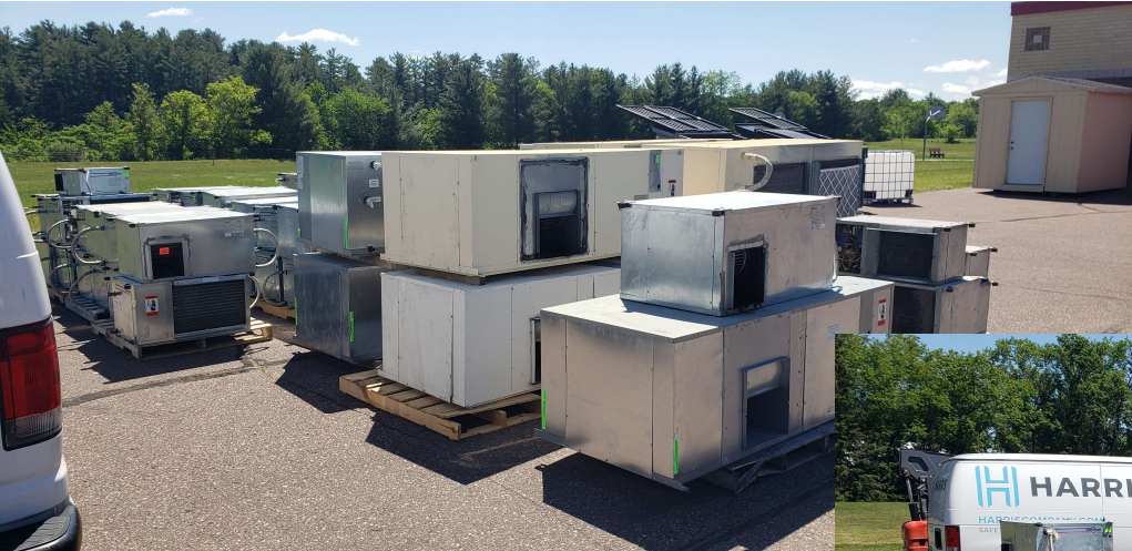
65 old heat pumps removed
