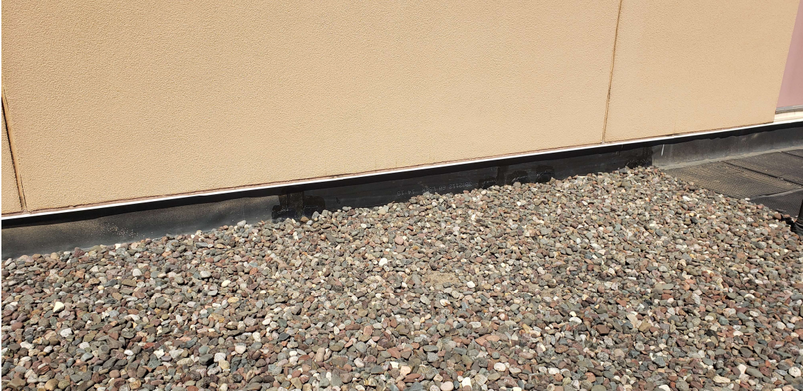
300+ feet of rubber membrane repaired on roof
